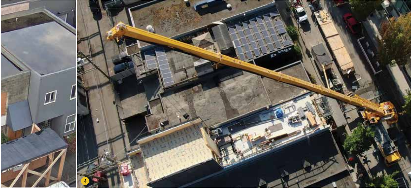
4. Virtual construction analysis also decided the selection of a crane that could reach from the street to the rear of the lot.
