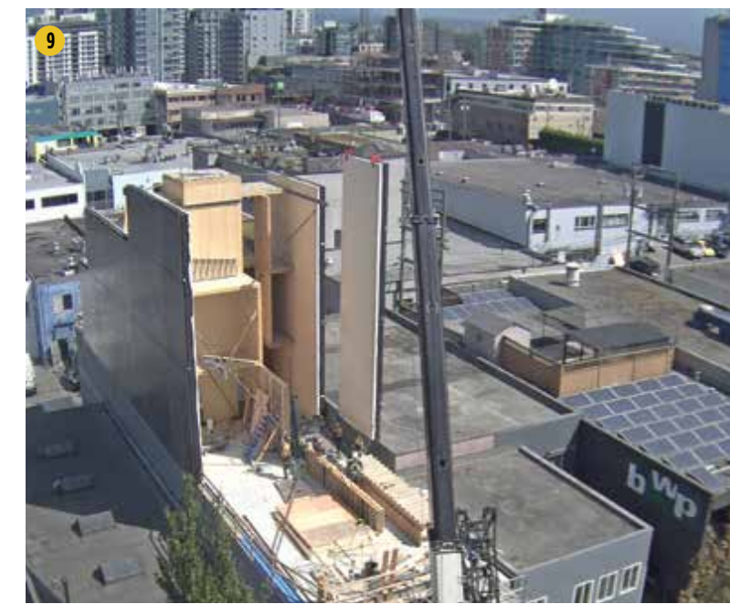
7. The project refined the virtual construction process in a series of meetings held over four months. 8 and 9. The virtual construction process also informed the choice to build the structure from front to back of the lot.
