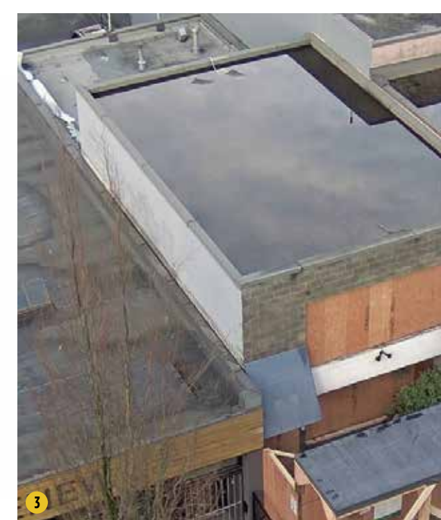
3. Virtual construction analysis showed that the optimal staging area to be the floor slab of level 2.
