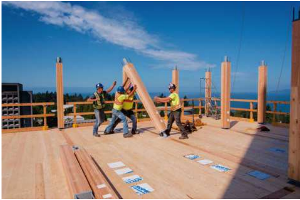
Glulam post installation
