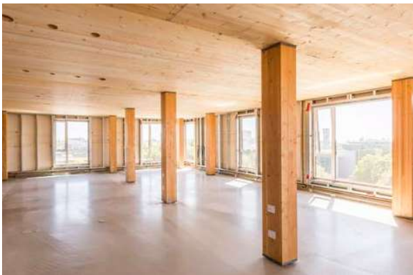
Residential floor interior prior to gypsum board encapsulation
