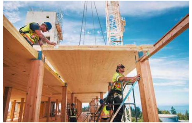
CLT panel installation
