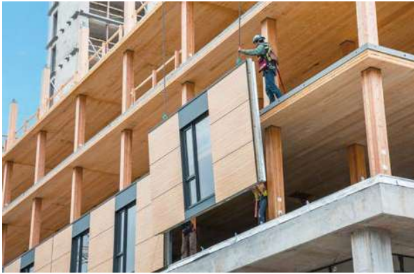
Glulam post installation
