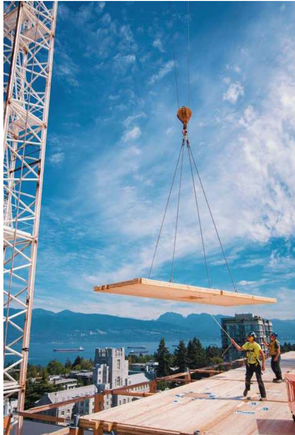
CLT panel installation
