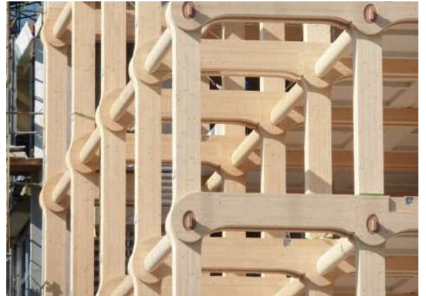
The joint configuration, combined with tapered diagonal members, enables the frame to resist twisting and bending.
