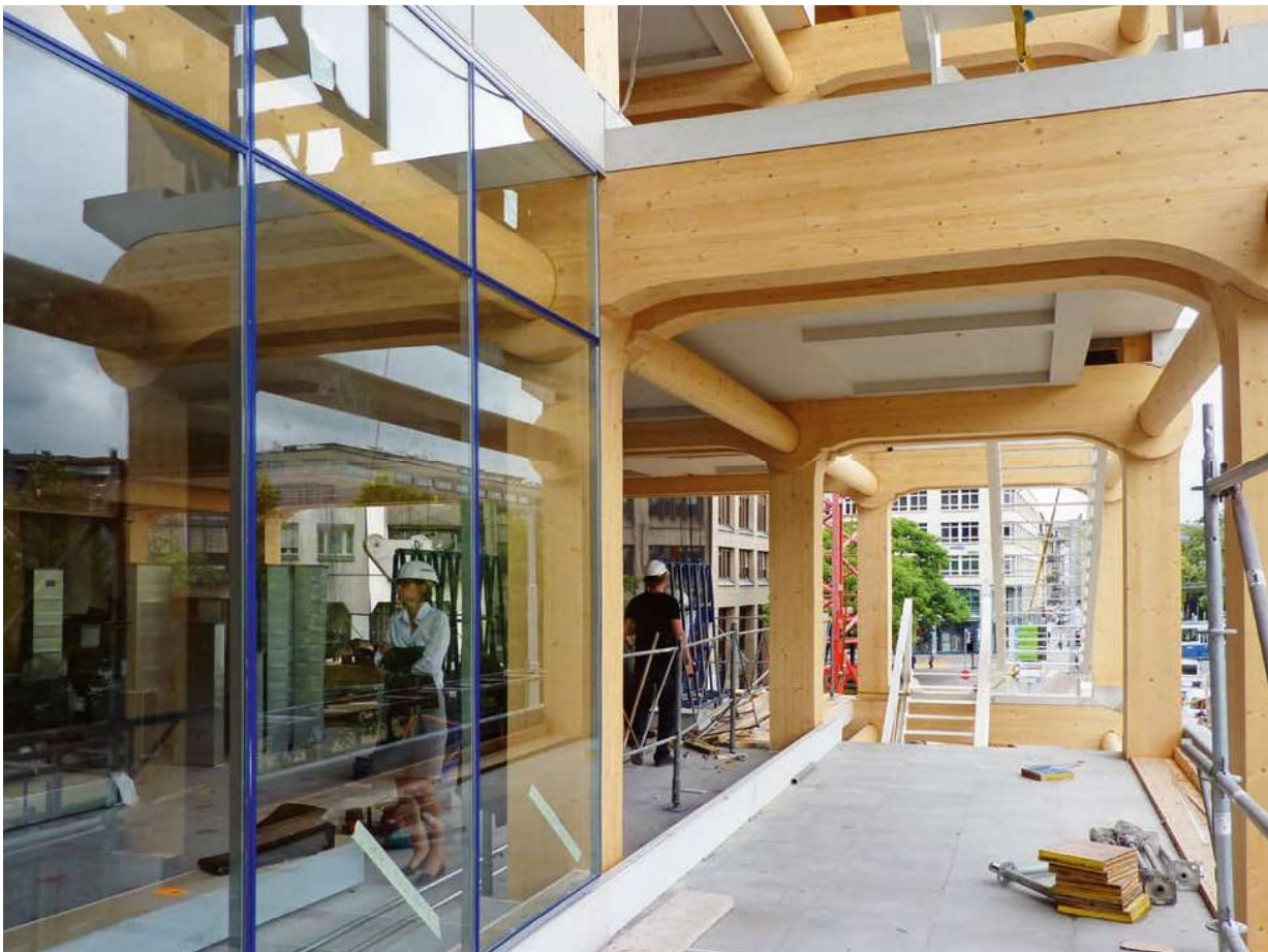
Components combine to create a unique and expressive post-and-beam system.
