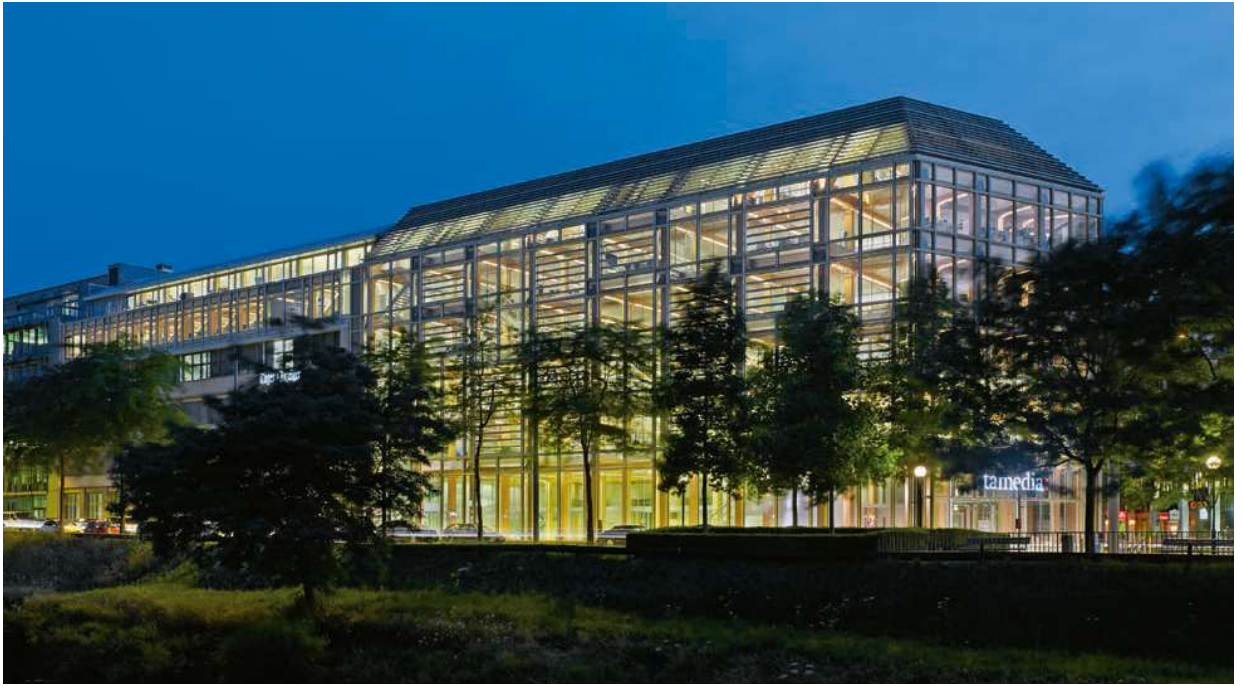
The structural rhythm and mansard roof form of the building responds to the historic context of the site. The new building extends over the adjacent building, creating meeting and office spaces.
