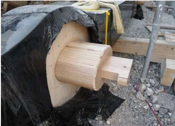
The joint configuration, combined with tapered diagonal members, enables the frame to resist twisting and bending.
