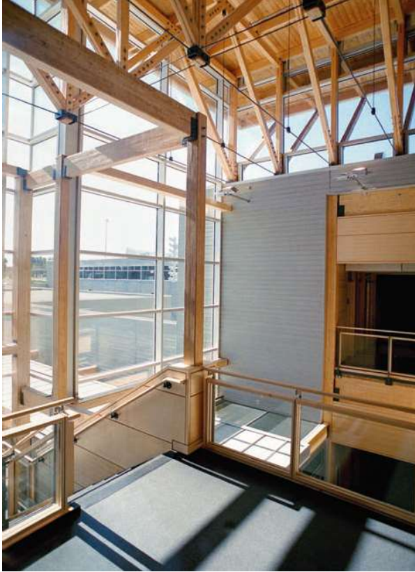
An analysis of the wood structure and finishes of the Eugene Kruger Building, Laval University, Gauthier Gallienne Moisan Architectes, 2005, in Quebec City, Canada demonstrated a significant reduction in embodied energy compared to a steel equivalent.
