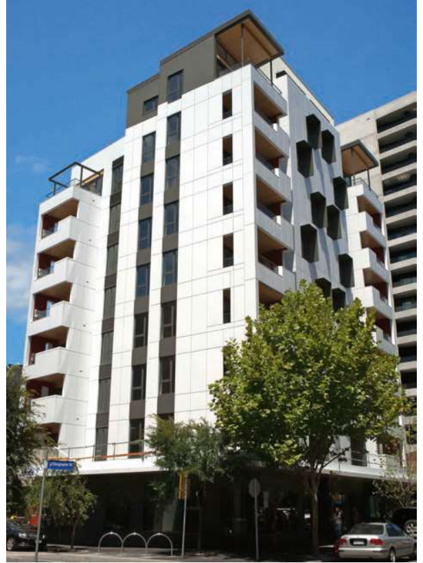
The imported solid wood structure of the Forte Building, designed by Andrew Nieland/Lend Lease Corporation and built in 2012 in Melbourne, Australia, has a lower carbon footprint than a similar structure built from local concrete.
